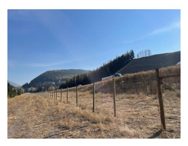
Image 6. Phase one wildlife exclusion fencing between Loop Bridge and Carbon Bridge.
