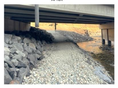
Image 5. Example of an underpass retrofit at Old Town. A similar approach to Alexander Creek was used on the NW side of the bridge, where a 1.5 m wide path was created through the large rip rap and filled with pea gravel to create a surface more ammenable to wildlife. The SE side of the bridge was already very open and serving as an underpass with no work needed. use.
