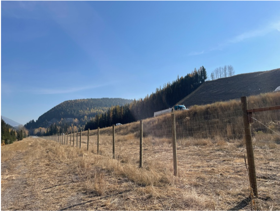
Image 4. Phase 1 wildlife exclusion fencing between Loop Bridge and Carbon Bridge.
