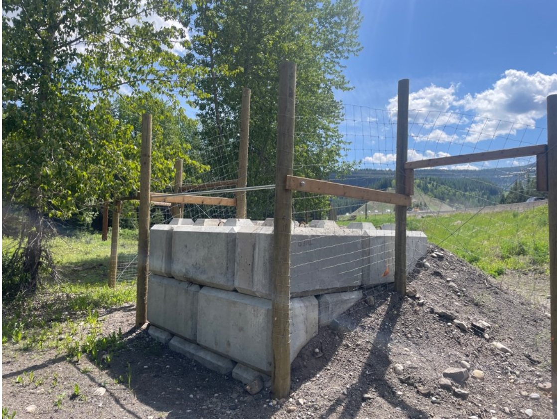
Image 5. A jumpout along the Phase 1 fence. The jumpout was designed based on extensive testing from Arizona using elk, bighorn sheep, and deer (Gagnon et al. 2020). This design is simple and allows animals to safely exit the highway if needed, while precluding animals from jumping into the highway right of way in reverse. Where sheep are a concern the grooves between the blocks should be filled. The horizontal bar at 45 cm above the exit ramp reduces animals jumping back into the right of way.
