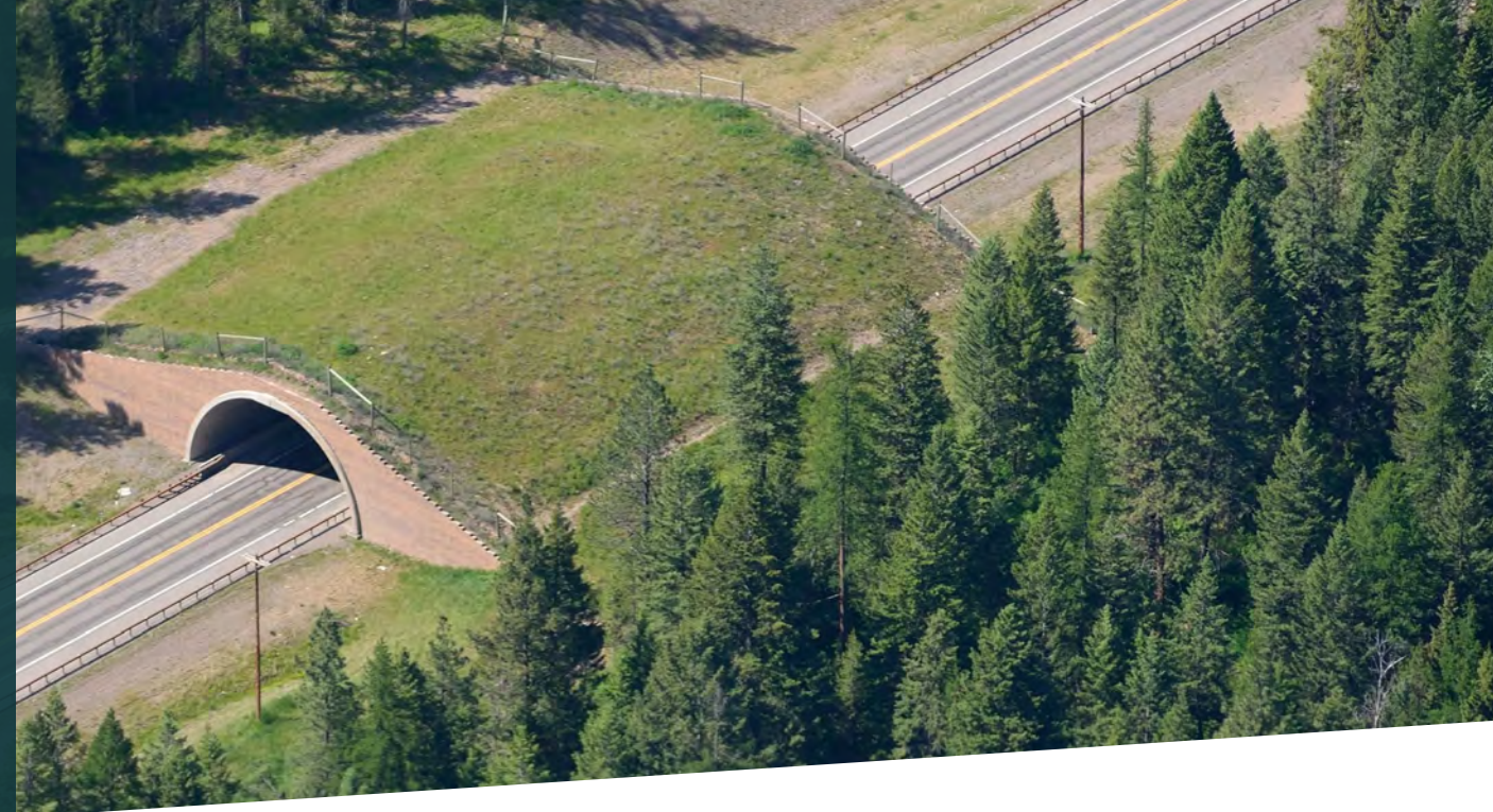
A wildlife overpass on Montana's US 93 is one of 41 fish and wildlife crossing structures built with Confederated Salish and Kootenai tribal knowledge. Photo credit: Marcel Huijser
